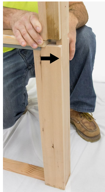
Flush aligned for rough opening
